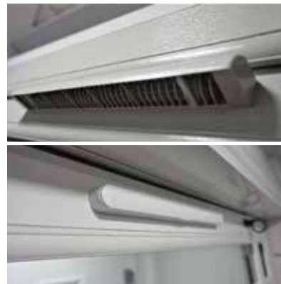
Trickle Vents Adjustable internal tumbler and external built in fly screen. Please speak to your installer about ventilation, current building regulations and how it affects you.
